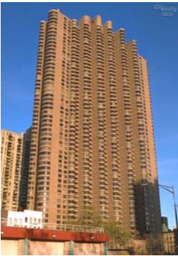
The Corinthian NY, NY. Central Chiller upgrade 2006, saving 778 KW per year.
